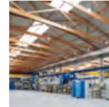
Glue-laminated timber is ideal for heavy-duty and long-span components. It has high strength and stiffness. It has high shape resistance and dimensional stability. Glulam's high carrying capacity is nearly 80 % that of wood, and can therefore reach any timber length up to 40 metres. In our competence saw center 32 metre-long glulam are used as supporting elements. This is also: *Materializing Excellence*.
